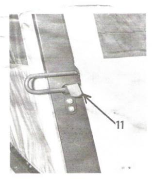
Insert ¼" x ¾" carriage bolts into door latches and put on lock washers and nut. Slide heads of carriage bolts into slots in uprights. Close doors and slide latch up under door handle so it puts a little tension on door. Tighten nuts. Place cap nuts over ends of bolts.
